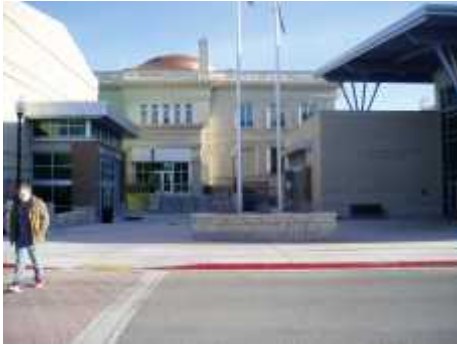
Elko County administrative offices and Court House Plaza
