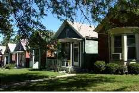
An older residential neighborhood that has been preserved and restored
