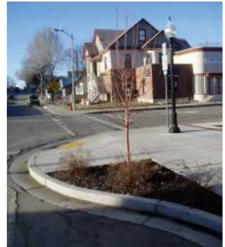
The curb extensions/returns above are located in downtown Elko. Curb extensions reduce the length of the crosswalk. They also calm traffic at intersections and can be good locations for landscaping
