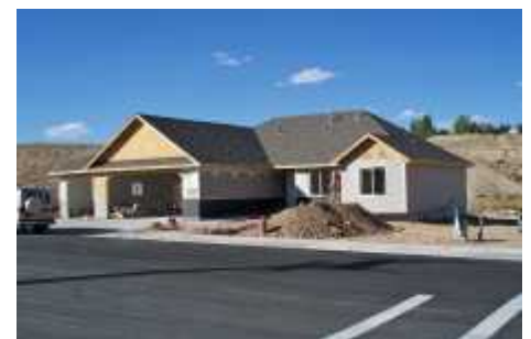
Single family home under construction in Elko's north central neighborhood
