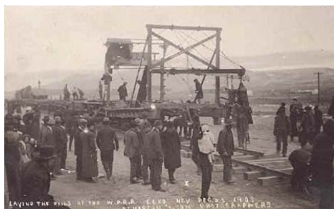
Western Pacific Railroad tracks being laid in Elko, December 1908. www.elkorose.com
